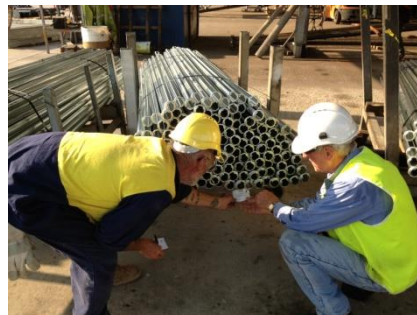
QA Inspection & Tag Recording
