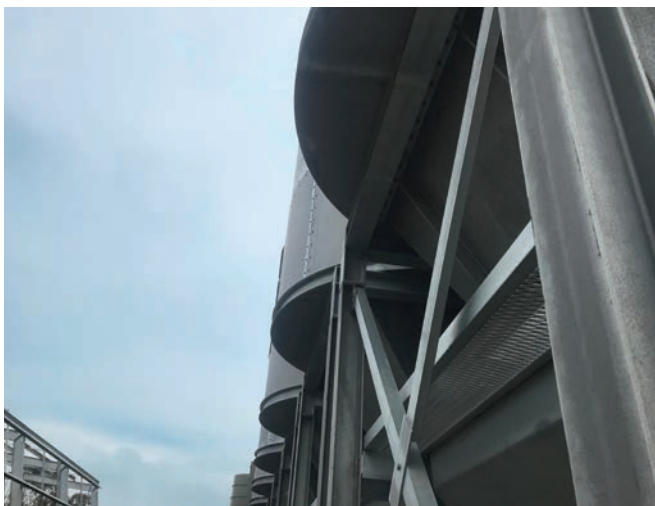
Boral CBD Concrete Manufacturing Plant, Victoria
