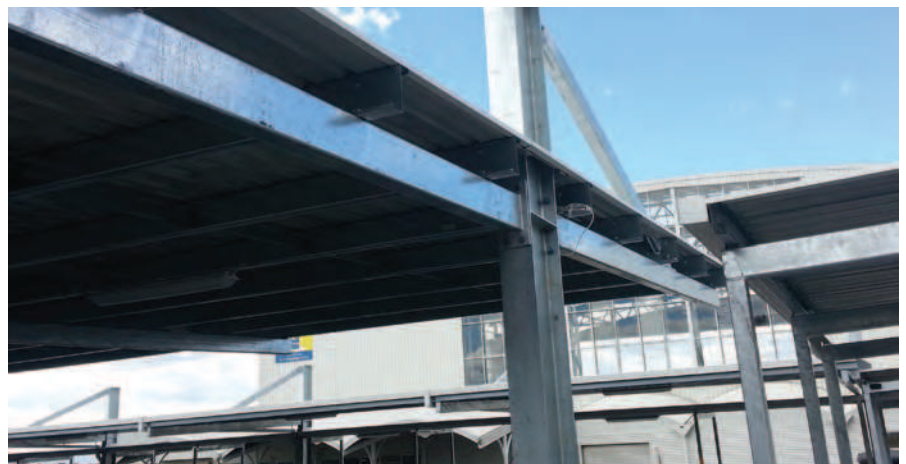
Figure 10: A car park structure with typical bolted connections
