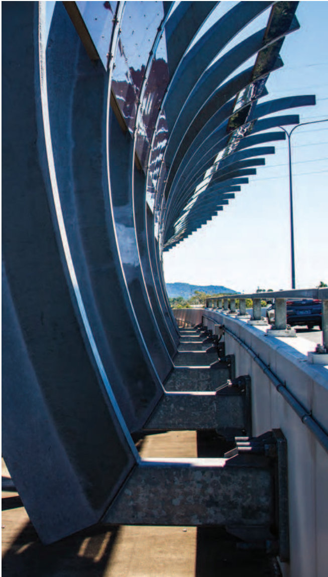
Figure 1: Roadside barriers come in all sizes and shapes, with this HDG crash barrier and sculpture bolted directly onto the concrete wall on this overpass in Queensland
