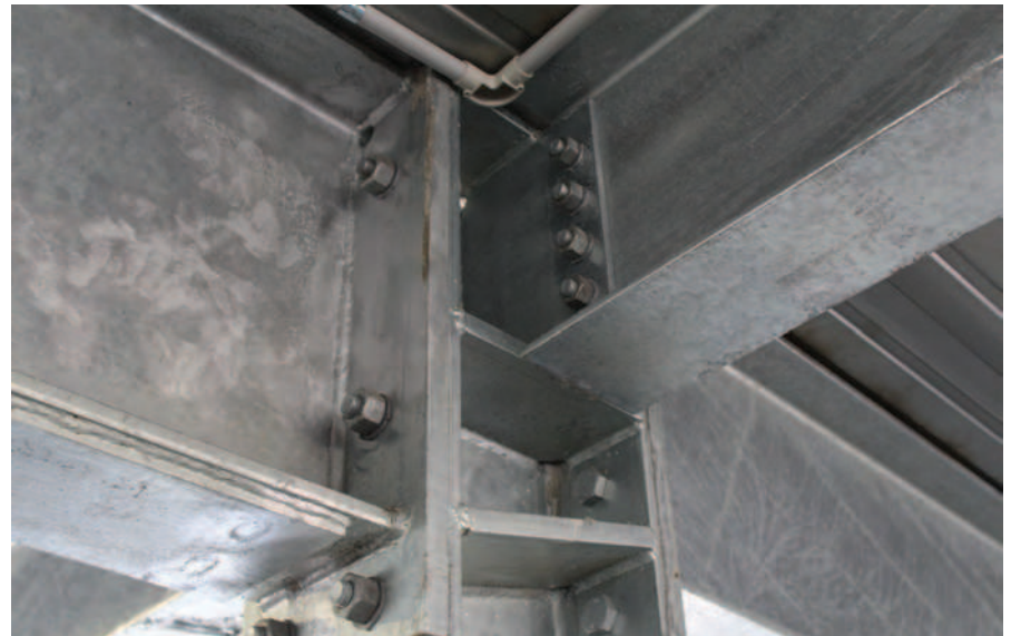
Figure 7: The Austin hospital carpark made extensive use of bolted connections for complex joints
