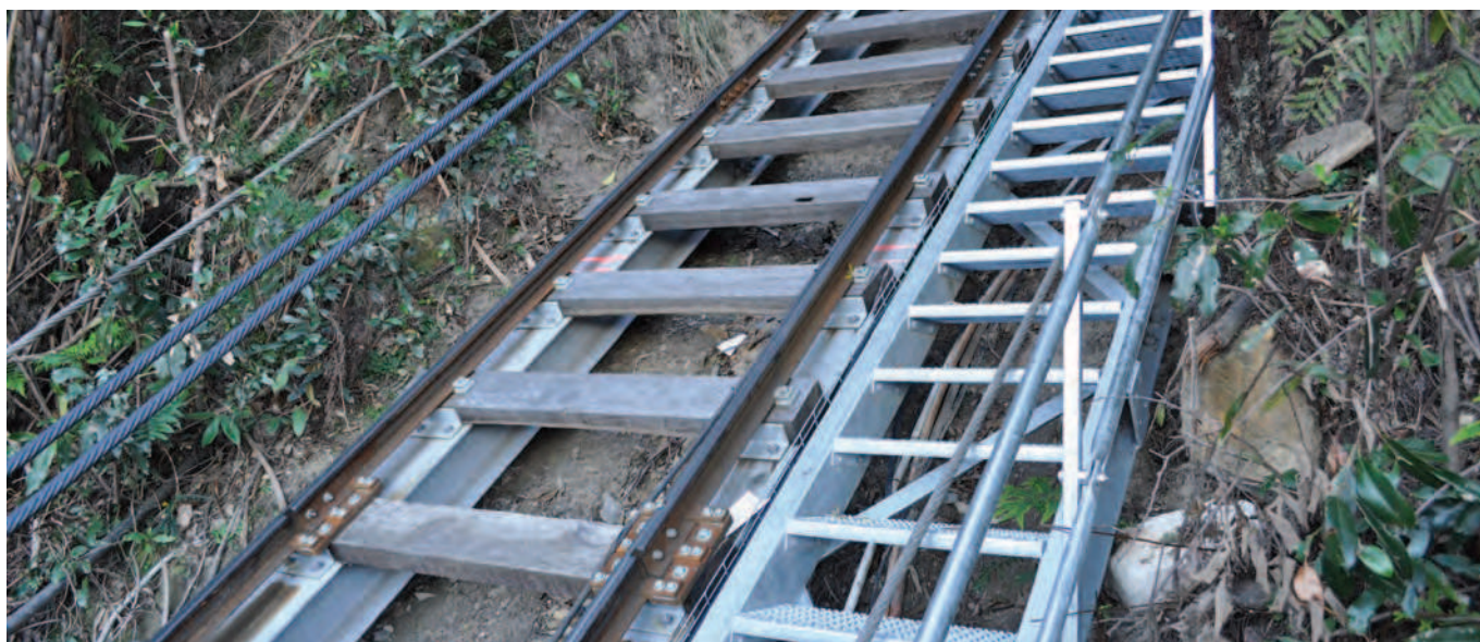
Figure 19: The Scenic railway in the Blue Mountains in NSW showing the use of HDG bolts in railway sleeper and stair connections
