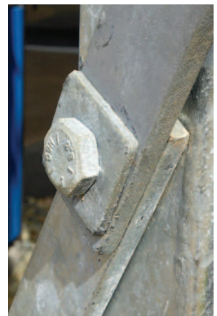
Figure 16: High strength bolted connection joining multiple plies
