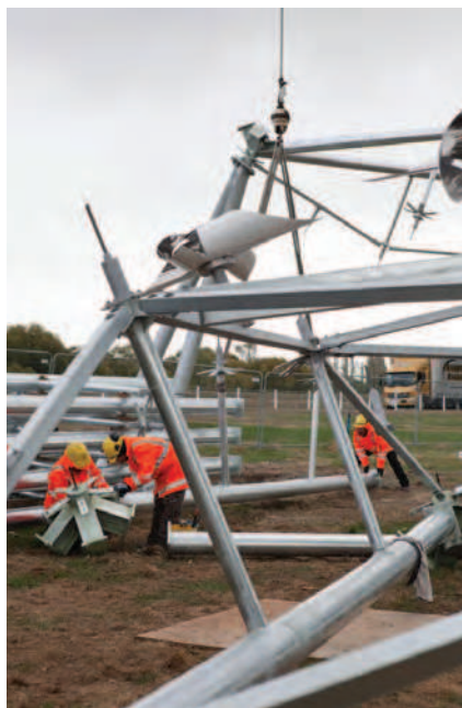
Figure 17: Modular construction is enabled through bolted connections
