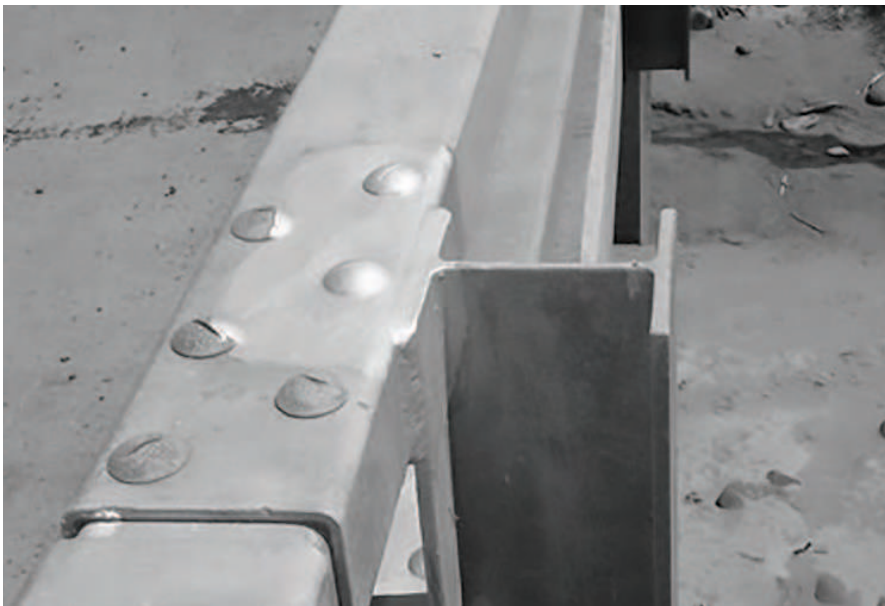
Figure 16 An example of a well repaired crash barrier in a severe marine environment
