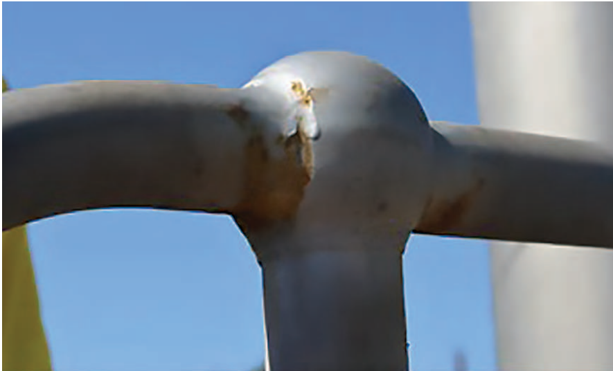
Figure 15 An example of poorly repaired handrail in a severe corrosive environment (wastewater treatment plant) where the repaired area has failed well before the main hot dip galvanized rails and posts
