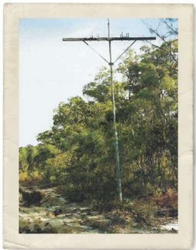
The original 1883 overland telegraph pole system was thought to have another 200 years of life left in the galvanizing when it was decommissioned in 1997.
