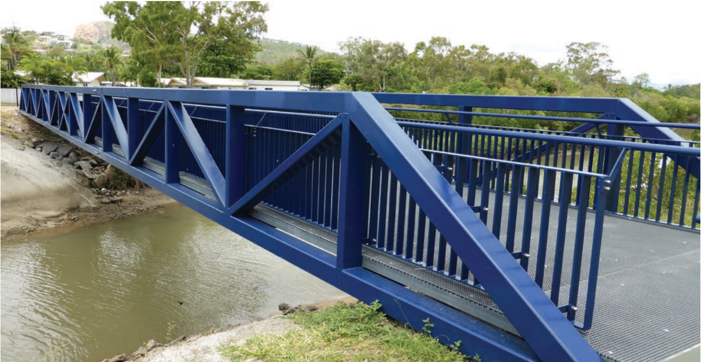
Figure 5: Duplex coated pedestrian bridge located at Captains Creek, Townsville, Queensland
