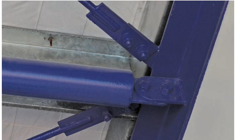
Figure 1: Close-up of some of the duplex coated structural members inside the Queanbeyan, ACT Pool after around eight years' service
